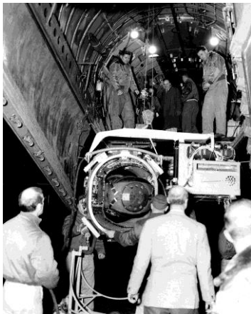
Figure 12. Spiire During B-29 Installation.
