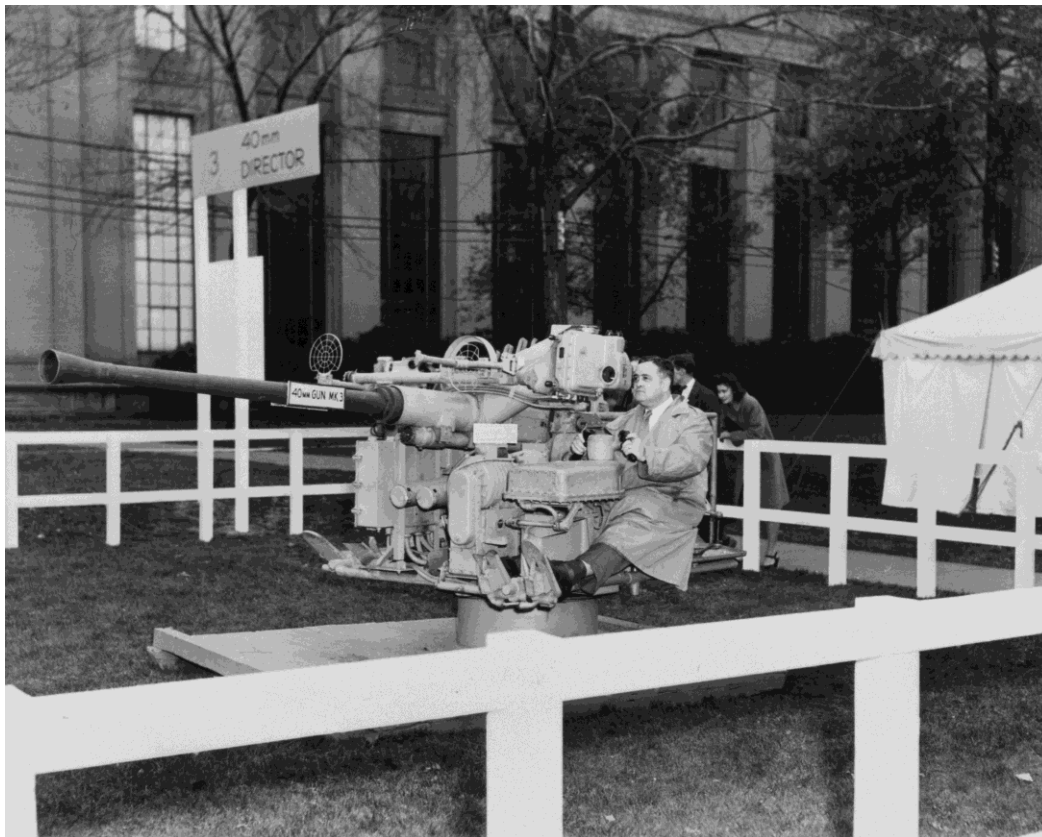
Figure 9. Draper Displaying a Naval Ship Defense Gun with an Integrated the Mark 14 Gunsight.
